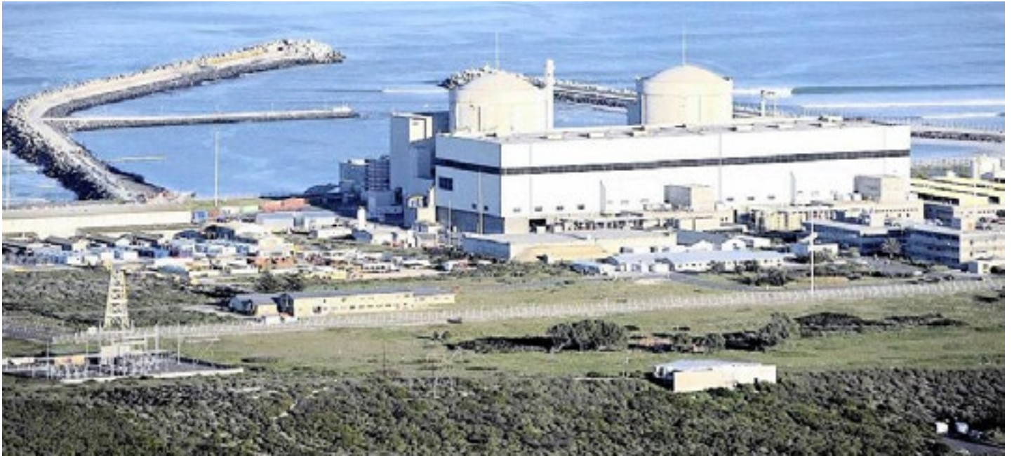
Koeberg power station
