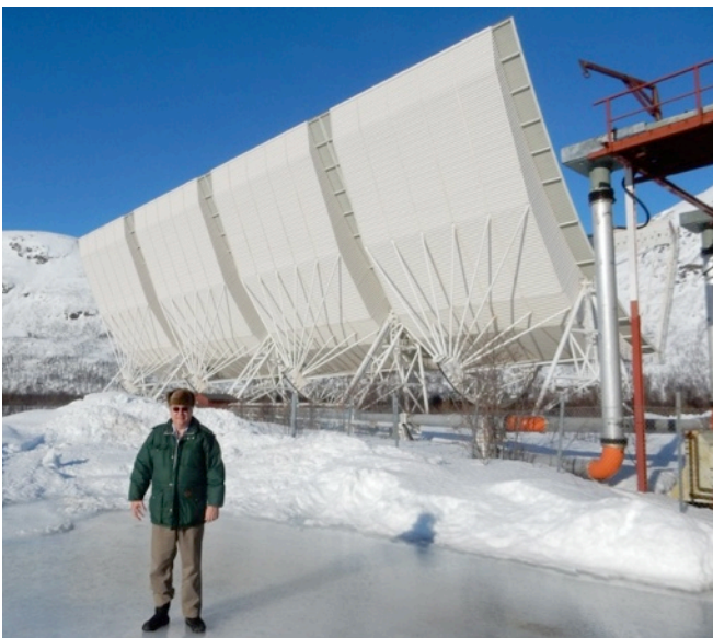
The EISCAT VHF radar near Tromsø in Norway is the largest radar of its type in the world, with a dish size of 120 x 40 metres.
