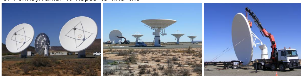
Figure 3: (left) 3 dishes in position. (middle) Fifth dish going up. (right) KAT-7 crane and dish.
