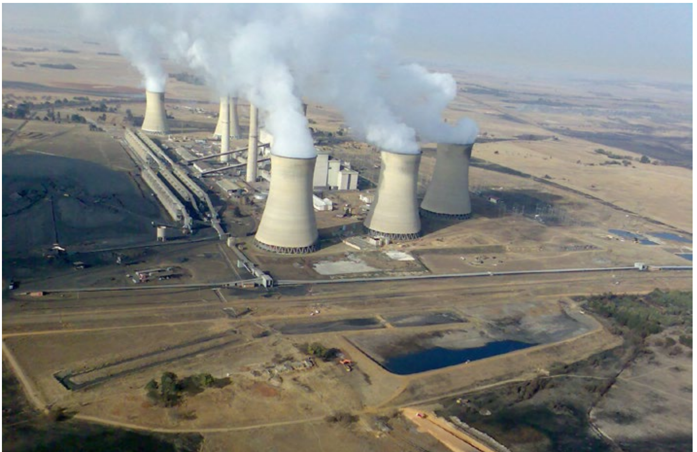
Arnot Power Station, Middelburg, South Africa (coal plant)
